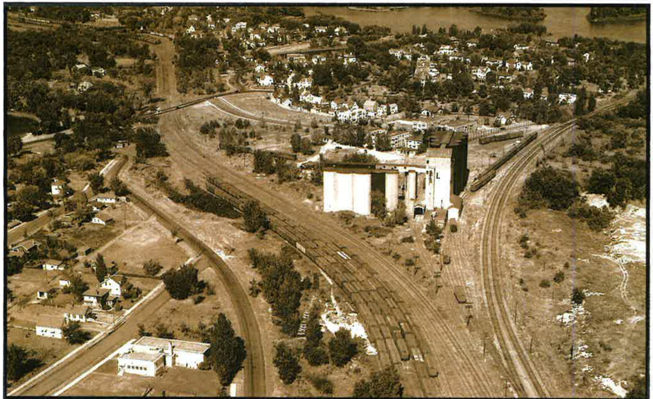
The Calhoun Isles condominium towers were built as grain silos in 1915 and 1928 and were converted to housing in the early 1980s. In this aerial photo taken in 1929 or 1930 by Joe Quigley, Lake of the Isles is at the top, with Cedar Lake on the left. The Minneapolis & St. Louis RR head off to the upper left through the Kenilworth Corridor. Alcott School (foreground), in service from 1921 to 1940, stands just west of Alcott Triangle near the intersection of West 29th Street and St. Louis Avenue. (Photo: Joe Quigley / Minneapolis Public Schools. Caption: Michael Wilson.)
